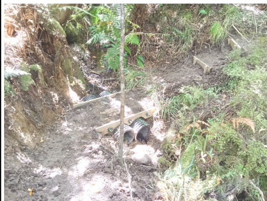
Earlier LandSAR challenges are now resolved by a ramped culvert pictured left
